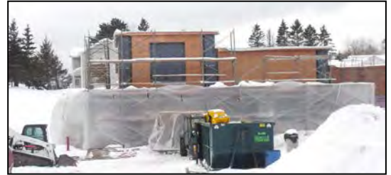
Aldi's under construction along Big Lake Road.
