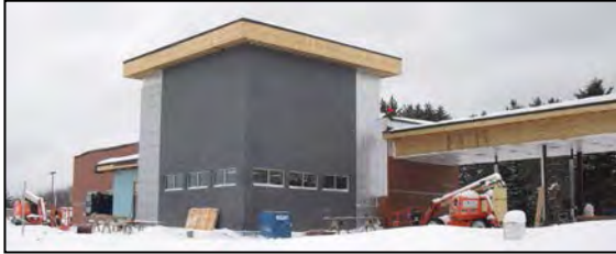
Members Cooperative Credit Union (MCCU) under construction along South Hwy 33.
