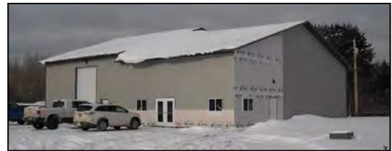
After a devastating fire in 2018 that yielded a total loss, Cloquet Interiors rebuilt on Hwy 33 North.
