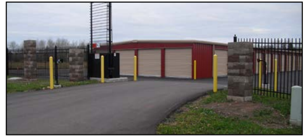
Building 2 and site improvements, Toy Barn Storage, Cloquet Business Park.
