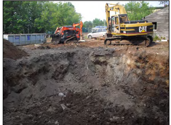
611 Adams Street demolition.
