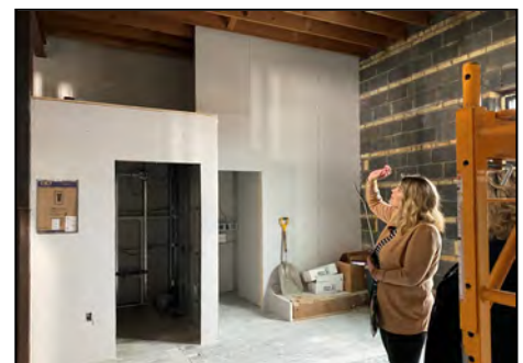
Union Lofts, loft construction progress photos.
