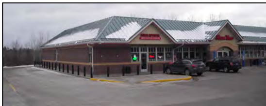
The City of Cloquet conducts inspections for the City of Scanlon, featured here is the building expansion and construction of a car wash in 2021 at the Hwy 45 Kwik Trip in Scanlon.
