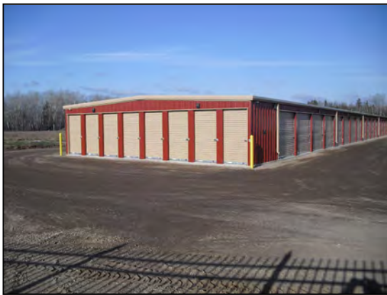
Third Toy Barn Storage Building in the Cloquet Business Park.
